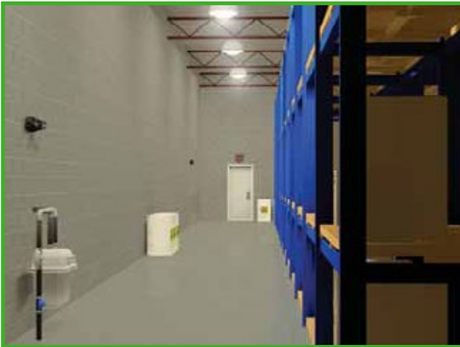
3D image showing installation of two TUF-NM Series battery units and a RNC combination unit in an industrial application under normal lighting conditions.
