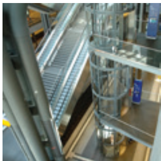
Elevators and Escalators
